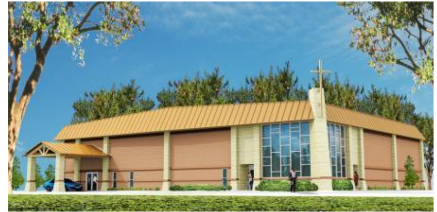
GLORY CHINESE BAPTIST CHURCH 3941 PARCHMAN ST. NORTH RICHLAND HILLS, TEXAS 76180 TERRY J. CUNNINGHAM ARCHITECTS 4000 W. UNIVERSITY BLVD., SUITE 1000, AUSTIN, TEXAS 78759
